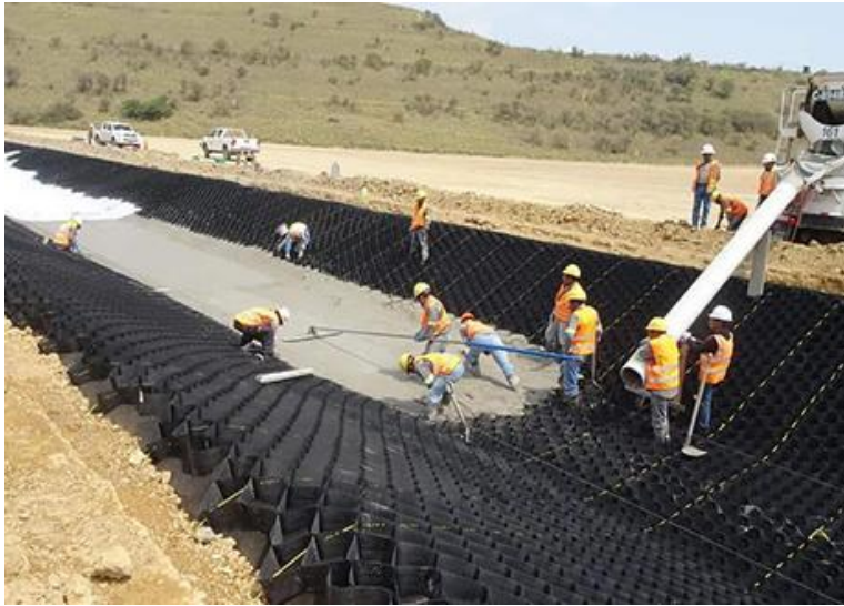
[Stabilize river embankments in Morocco]
