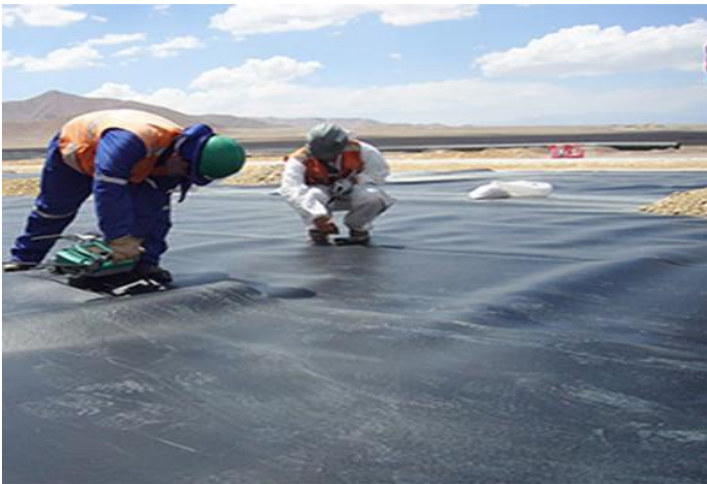
[Landfill in Ecuador]
