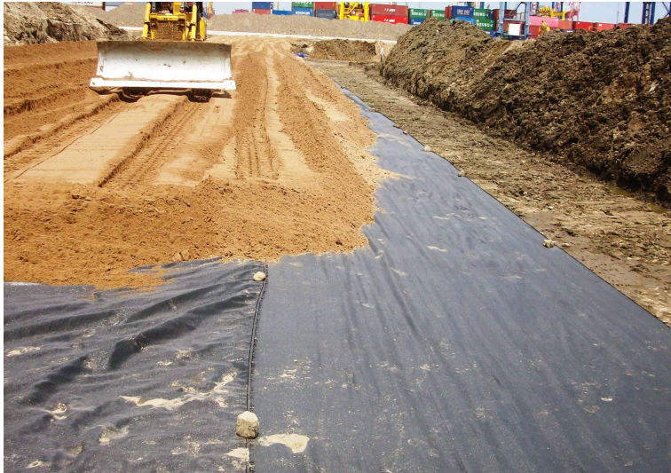
[Soft Foundation Consolidation in Philippines]
