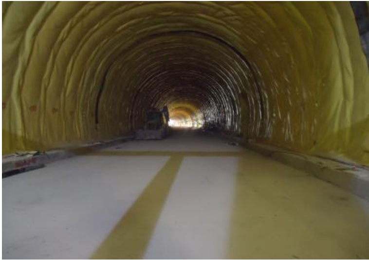
[Tunnel in Ecuador]
