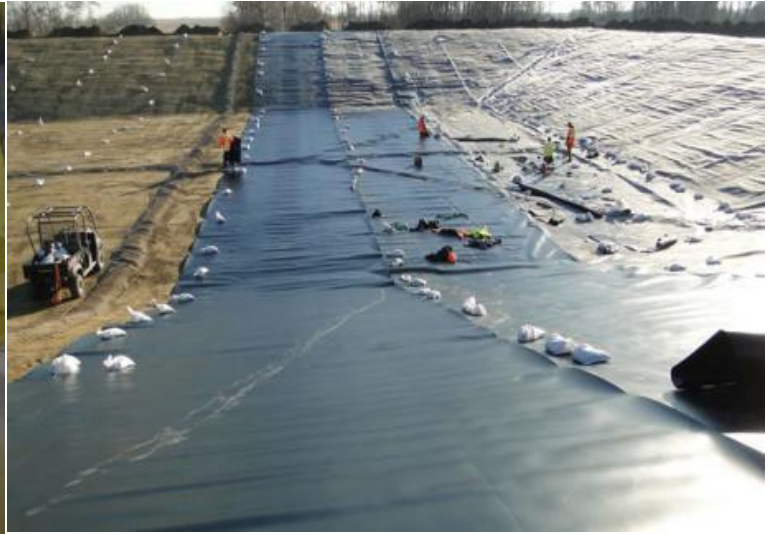
[Sewage Treatment System in Mexico]
