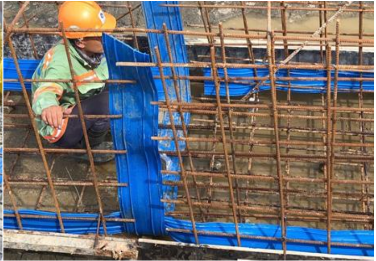
[ External Wall in Jordan]
