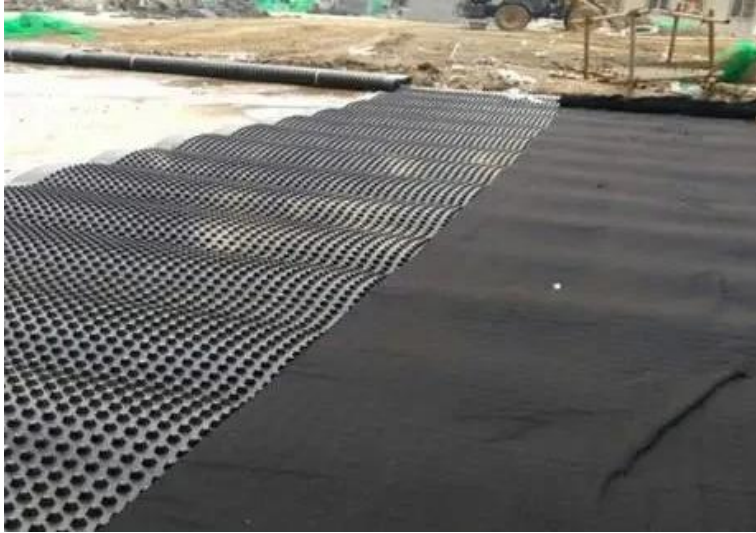
[Roadbed Drainage in Tanzania]
