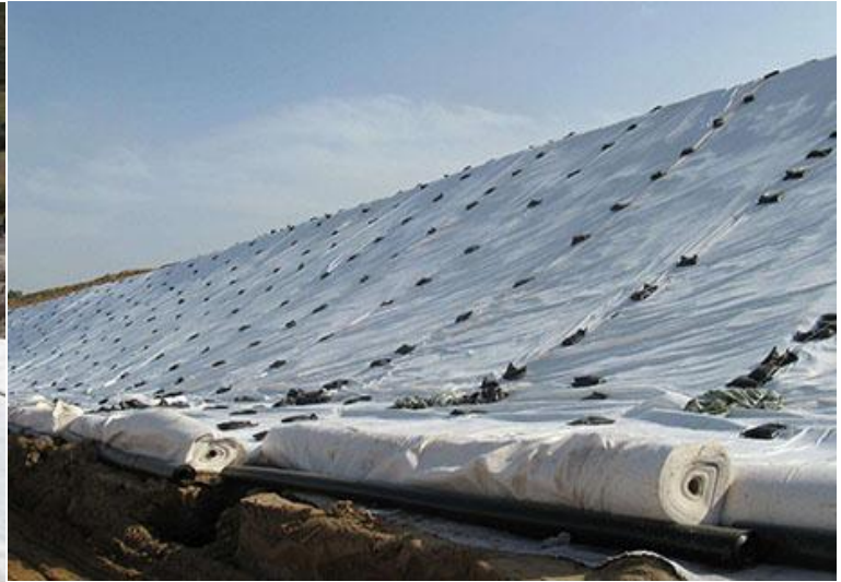
[Slope Protection in Finland]
