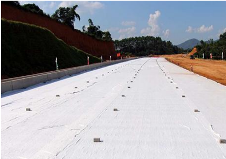
[Road Construction in Spain]
