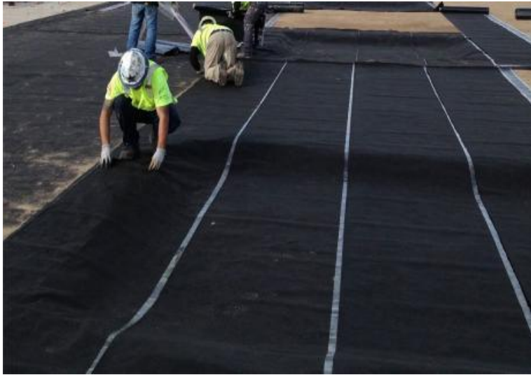
[Highway Waterproofing in Maseru]
