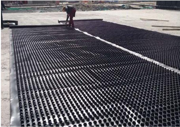
[Road Subgrade Engineering in Belgium]
