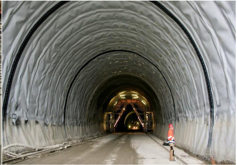
[Tunnel in Senegal]
