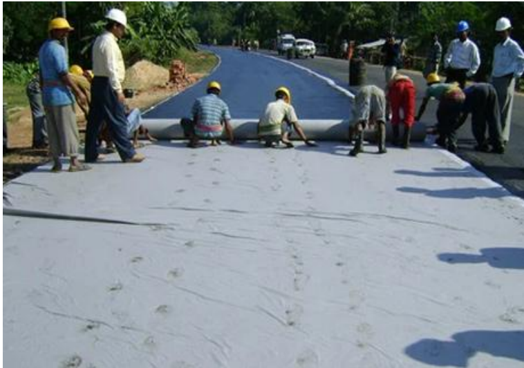
[Highway subgrade in Colombia]
