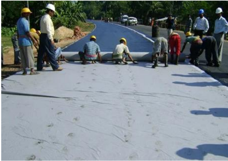
[Highway subgrade in Colombia]
