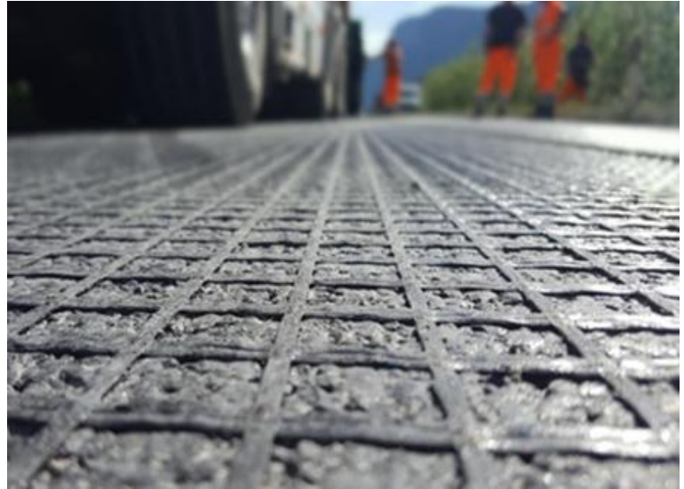
[Parking lot foundation reinforcement in Guinea]
