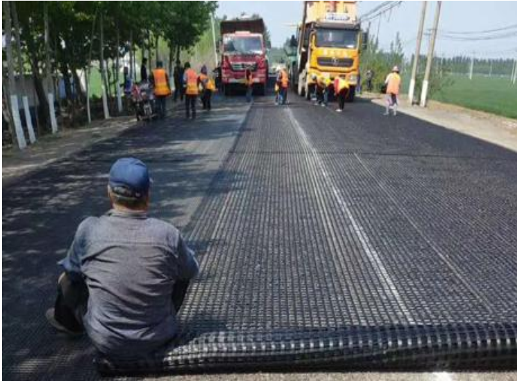
[old road reconstruction in Egypt]
