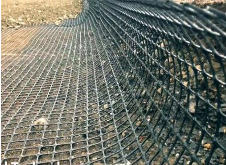
[Foundation reinforcement in Algeria]
