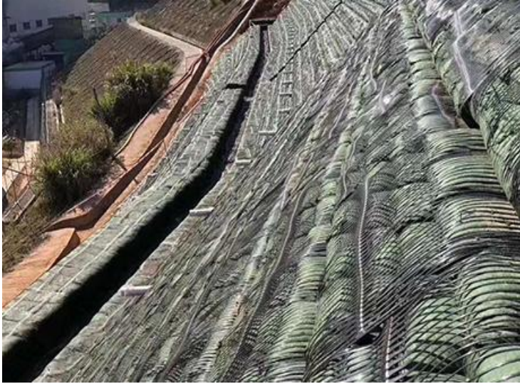
[Dam reinforcement in Rwanda]
