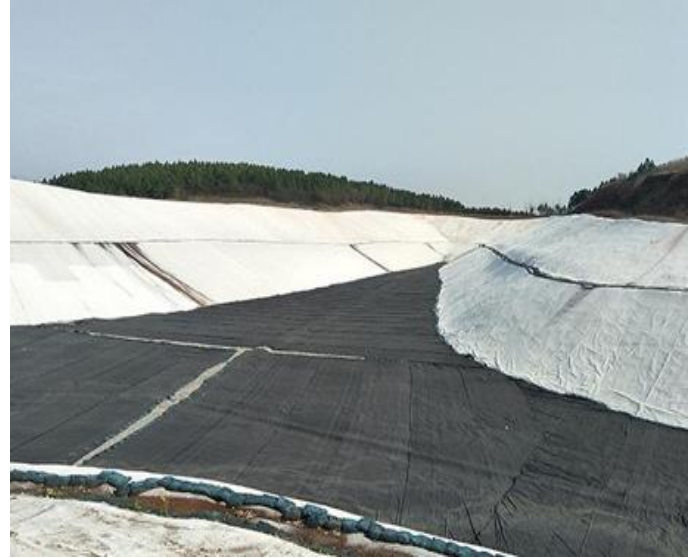
[Anti-seepage and reinforcement of water conservancy dams in Indian]
