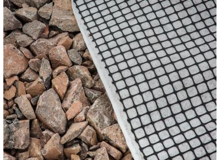
[Railway subgrade reinforcement in Ghana]
