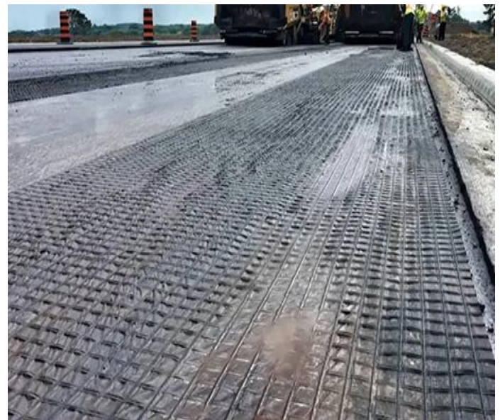
[Reinforcement of expressway in Senegal]
