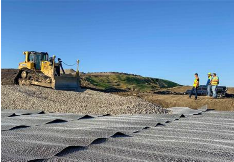
[Highway subgrade reinforcement in Liberia]
