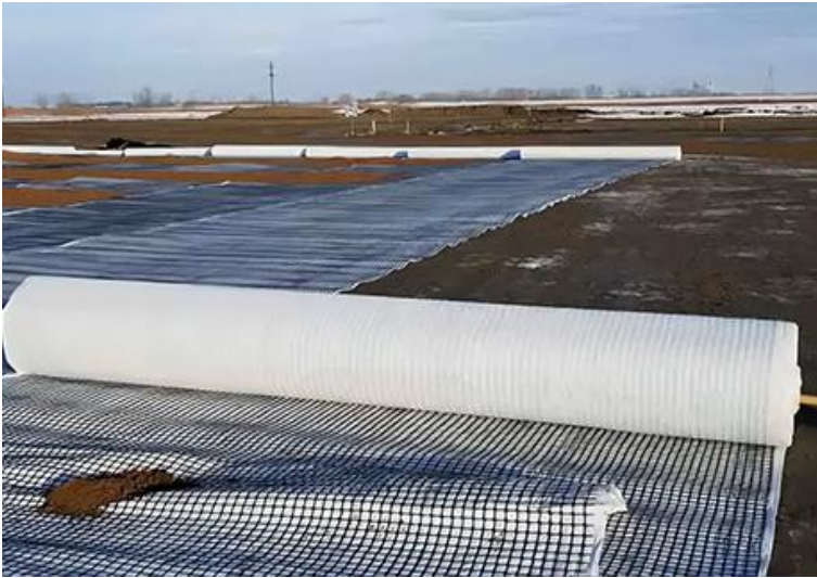
[Airport subgrade reinforcement in Sudan]
