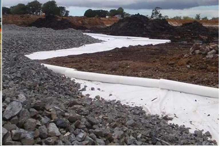
[Tailing Dam in Argentina]
