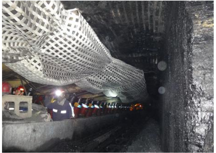
[False roof support for coal mine working face in Ethiopia]
