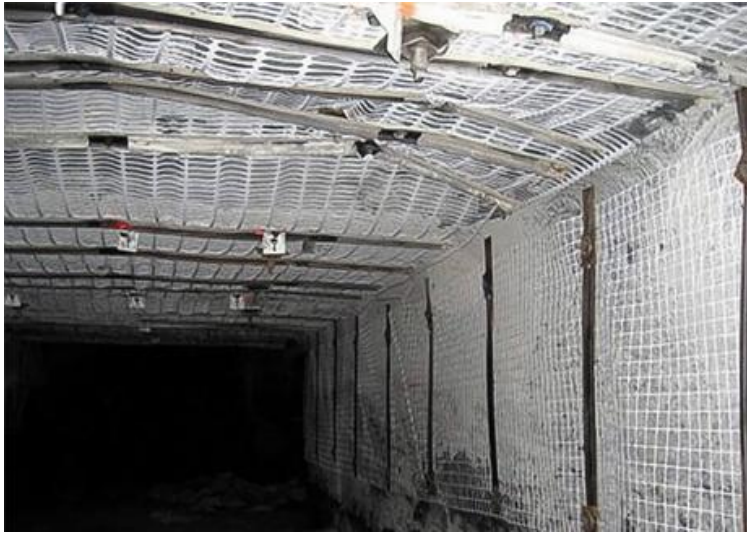
[Tunnel protection in Uganda]
