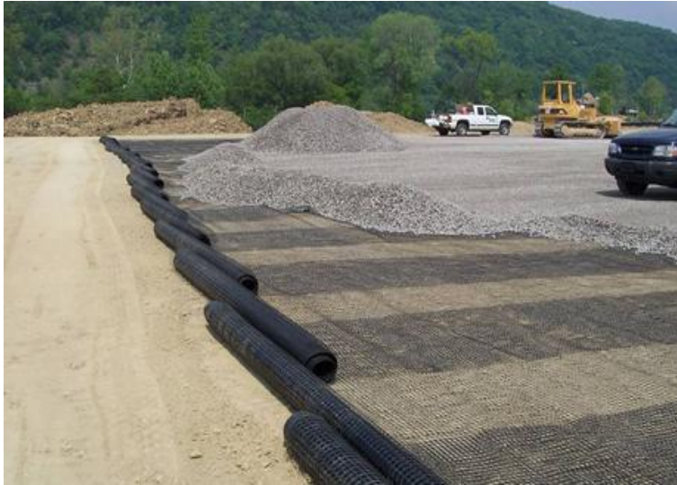
[Reinforcement of soil foundation in Ghana]
