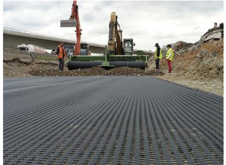
[Reinforcement of railway soft soil foundation in Tanzania]
